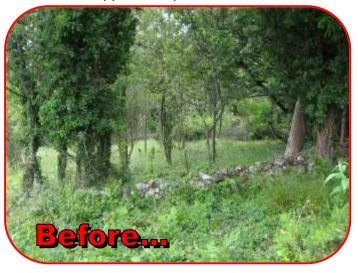
which was an ideal candidate for restoration, having safe access and being well away from the road. The wall was probably at least 200 years old and much of the stone had fallen down on both sides so that it was half its original height. It was also very distorted by tree roots and ivy.
