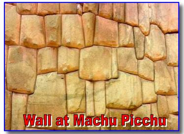
very resilient structures, even to earthquakes as the 600 year old Inca dry stone walls at Machu Picchu, Peru clearly demonstrate.
